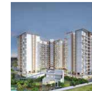
REGENCY ORION Baner Pune
