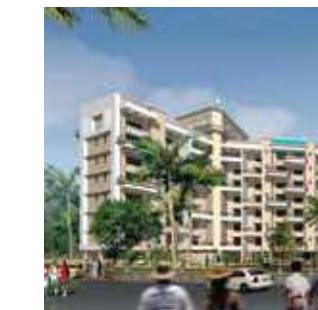
REGENCY ROSELAND Talegaon, Pune
